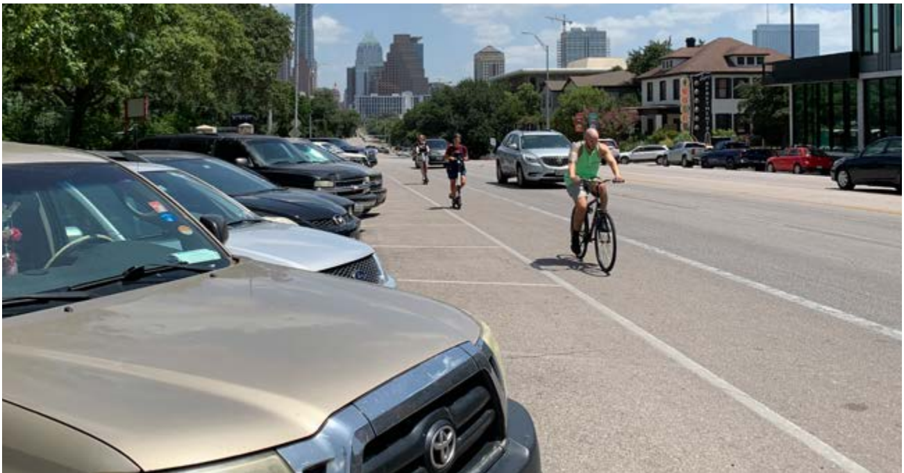
At night, many of these conflicts and safety challenges are amplified by dim or intermittent lighting along South Congress Avenue.
