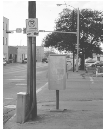
Utility equipment conflicts with pedestrian movement
